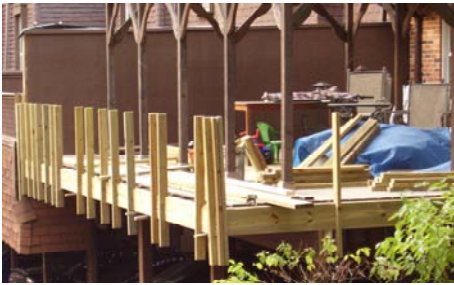
(The Wheeler's deck walls required complete replacement )
