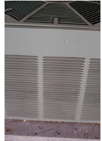
This type of unit is difficult to clean without removal of louvered cover
