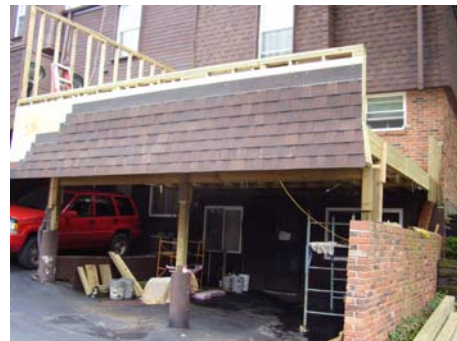
(complete deck replacement)
