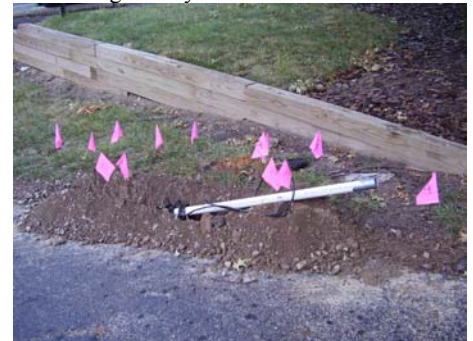
(water system under construction)
